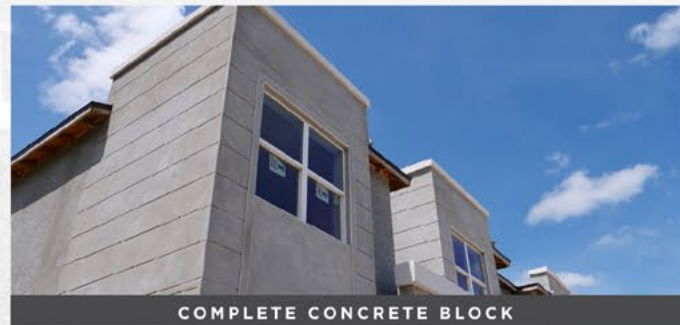
COMPLETE CONCRETE BLOCK
